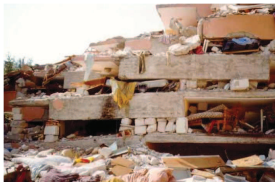
Figure 3 ► Pancake Collapse
